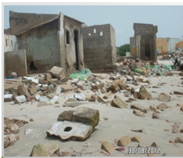
Figure 14: Debris du village DBD
